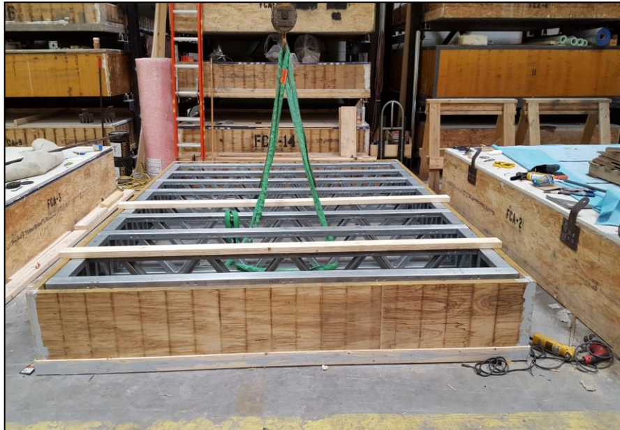
Construction of Test Specimen
