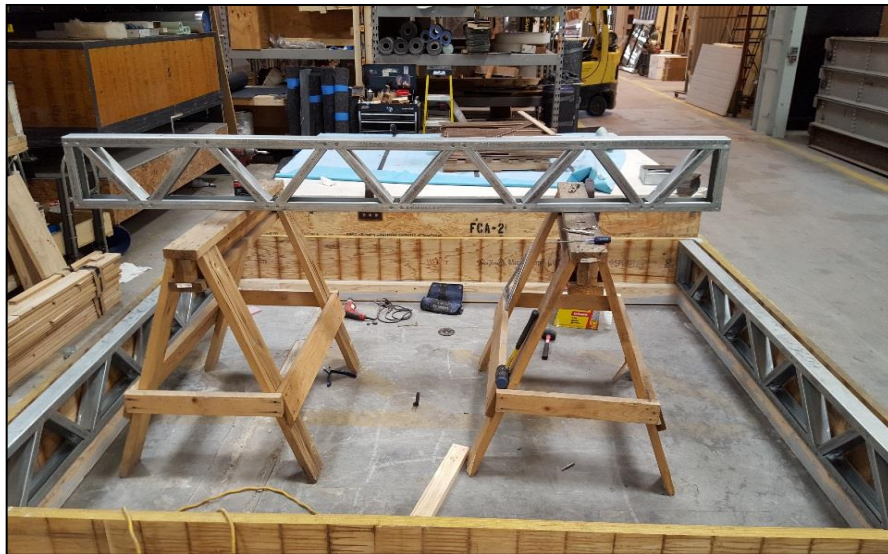
Construction of Test Specimen
